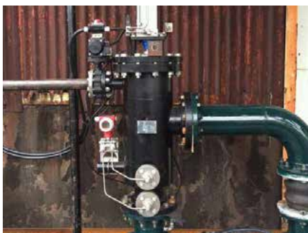
A Bernoulli Filter serves as a circulating cooling filter in the steel mill.
