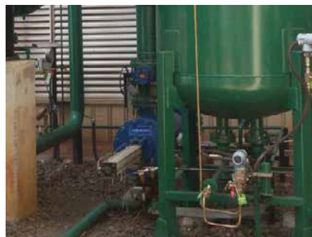
A Bernoulli Filter in a circulating cooling system removes suspended solids from the cooling water.
