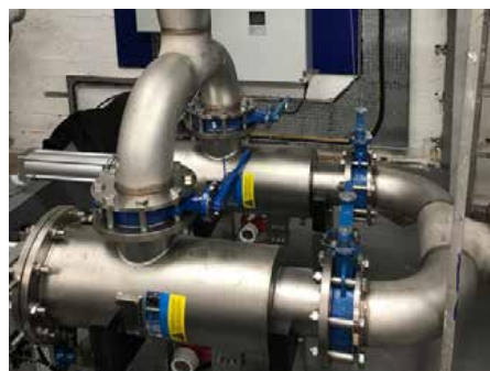
Two Bernoulli Filters are installed before a UV sterilizer in the aquaculture industry. They remove suspended particles from the water.
