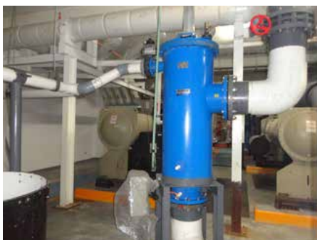
A Bernoulli Filter in a district cooling system removes the debris and particles, protects the tubular heat exchanger from clogging and improve the heat exchanging efficiency.
