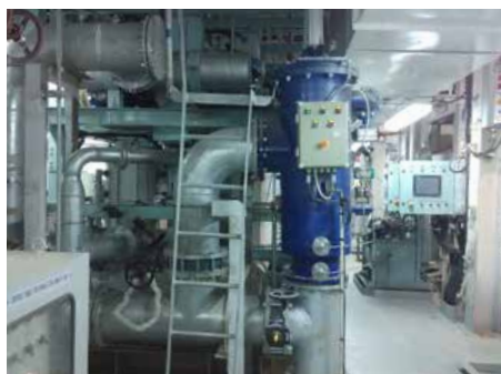
A Bernoulli Filter is working in a ballast water management system. It protects the downstream system from clogging.
